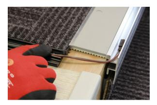
13. Cut the circuit board to required length.
