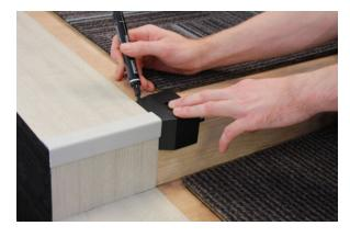
3. Measure between the back of the end cap that you have just marked on the tread to the front edge of the tread.
