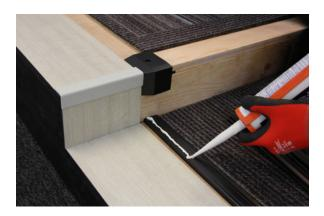
9. Measure the width of each step from end cap to end cap, or end cap to the wall and cut the step profile appropriately along with any backing plates.
