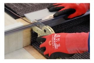
16. Insert lighting circuit into the PVC tube ensuring the lighting tube strip is facing the correct way. Insert tube into stair nosing.
