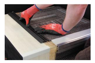
23. Install end caps, inserting the lugs into the appropriate retainers.
