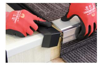
22. Secure the end cap with a screw and place the pip to cover the screw head.
